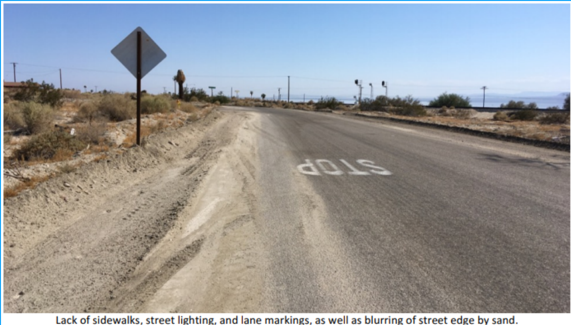
Lack of sidewalks, street lighting, and lane markings, as well as blurring of street edge by sand.
