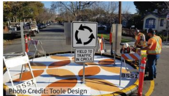
Quick-build traffic circle that could later be converted to a permanent design
