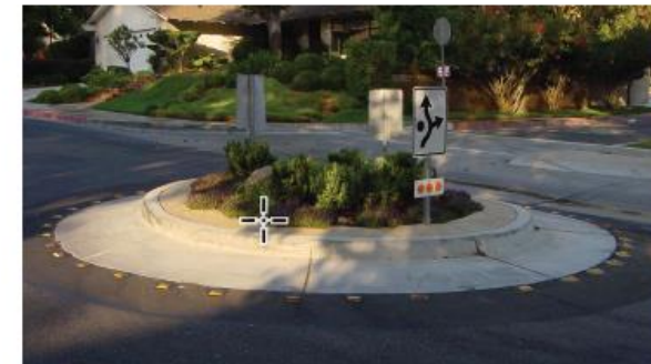
Traffic circle built with permanent materials with plantings
