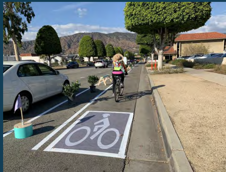
Example of separated bike lane
