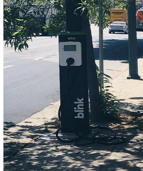
FIGURE 32. SAMPLE CURBSIDE EVCS
