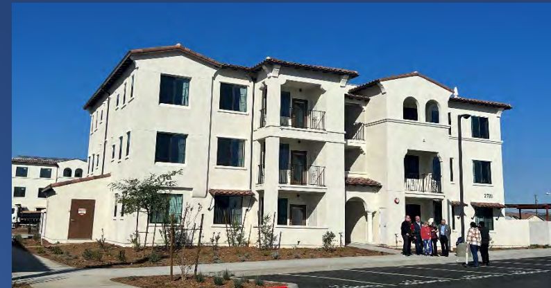
Somis Ranch Phase 1, Completed (200 units), Photo: Dec 2023
