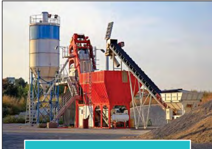
Concrete Batch Plants
