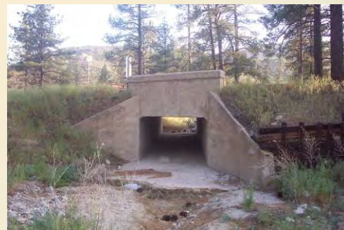
Example of a concrete box culvert on Highway 74 in Garner Valley.
