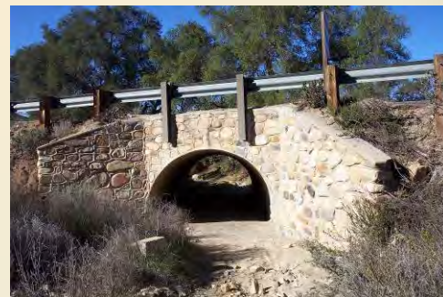
Kolb Creek bridge on the SR-79.
