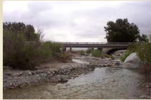
One of two bridges for Mission Creek; this is the southernmost bridge.
