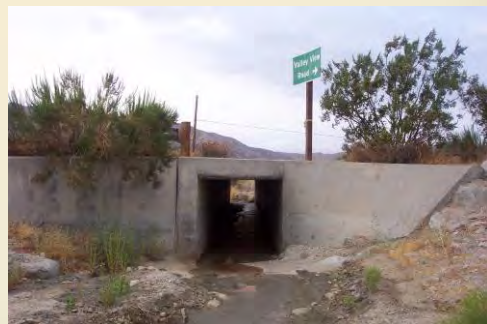
The culvert for Big Morongo Wash flowing under State Route 62.
