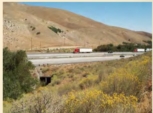
Culvert on Interstate-5 for Gorman Creek with Hungry Valley State Park in the foreground. Note steep degraded slopes on far side of I-5.
