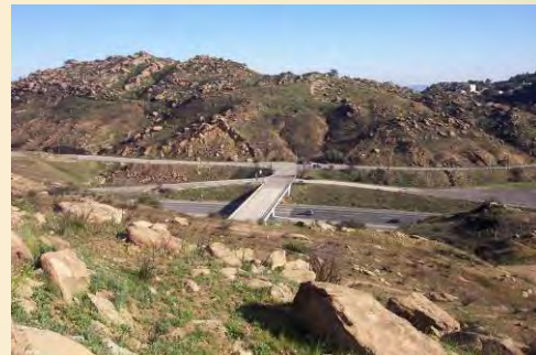
Looking south at the Rocky Peak overpass.
