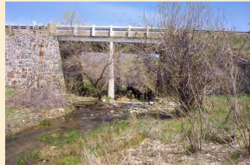
Bridge for Santa Ysabel Creek on SR-79.
