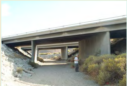
The north side of SR-58 at Sand Creek.
