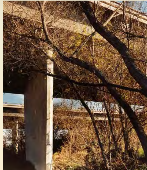
Temecula Creek passing through two extended bridges on Interstate 15.
