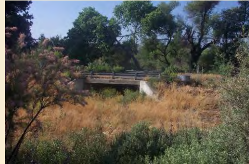
Looking up Tule Creek at the concrete box culvert under Highway 79.
