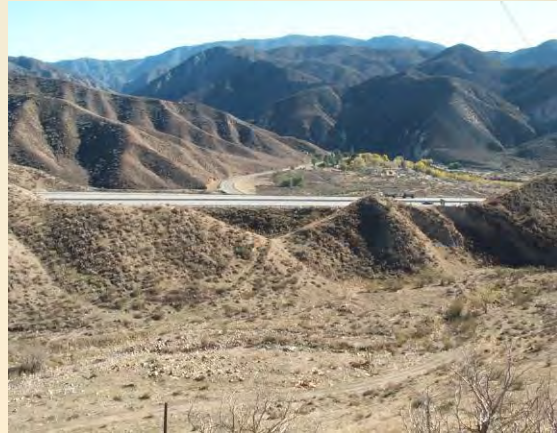
Removing the fill slope under SR-14 would route Spring Canyon to Bee Canyon and the Santa Clara River.
