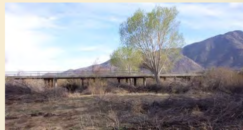
San Felipe Creek flows beneath SR-78 through a bridge that provides passage to numerous species.
