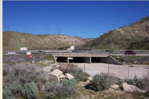
Gorman Creek undercrossing just south of I-5/SR-138 interchange.
