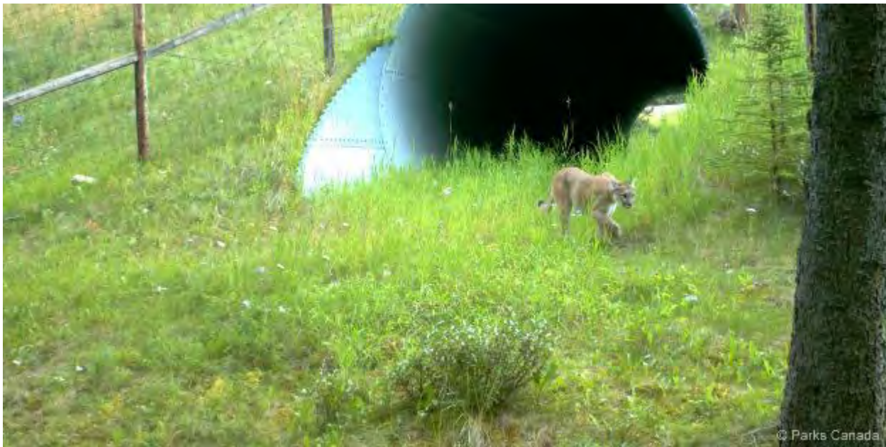
Mountain lion using a culvert. Photo credit: Parks Canada.
