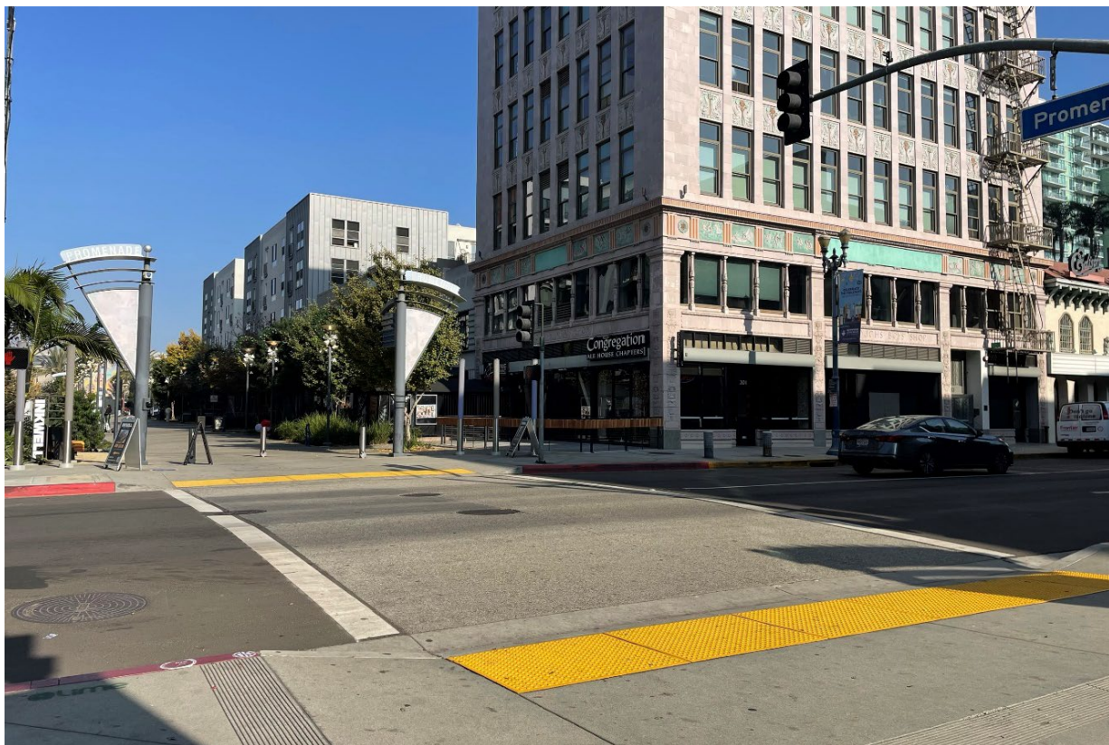
Exhibit 4 Pedestrian crosswalk in downtown Long Beach with APS and curb ramps.
