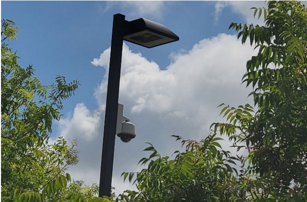
Exhibit 21 CCTV camera at Buena Park Metrolink Station.
