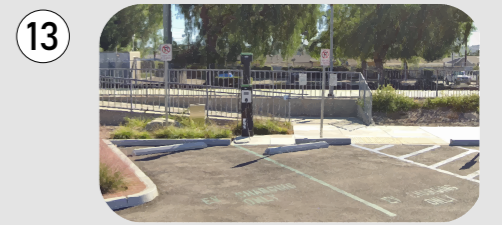
Moorpark Metrolink Station. Source: Google Maps
