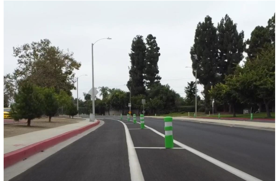
Merrimac Way, After
