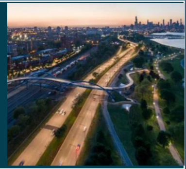
41 st Street Bridge (Chicago, IL)
