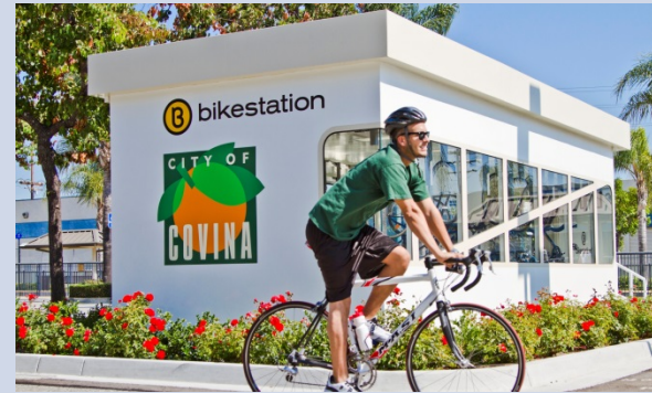
Secure Bicycle Facilities – BikeStation in Covina
