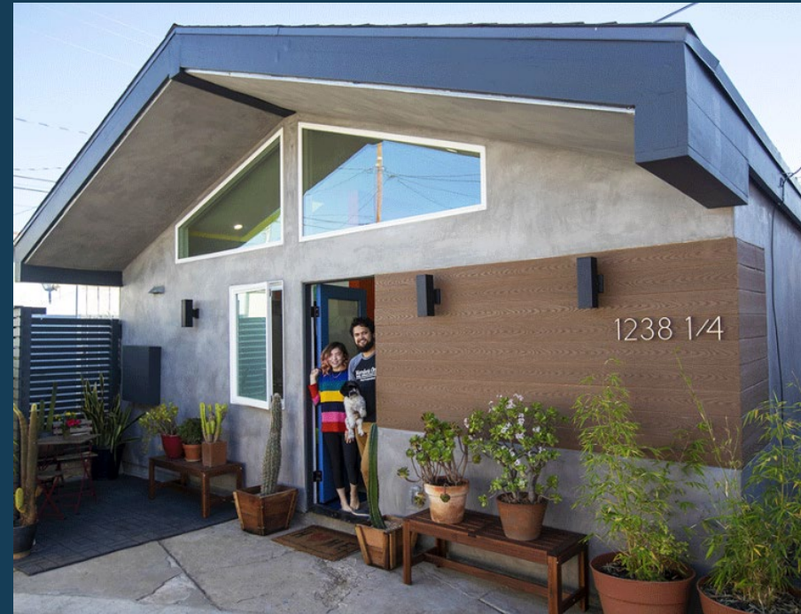
“Casita L.A.,” a new ADU in East L.A. designed by Alexis Navarro in carport area. “He challenged himself to build an ADU for under $100,000. What’s his secret?”, by Lisa Boone; Photo by Allen J. Schaben / Los Angeles Times, March 18, 2021.
