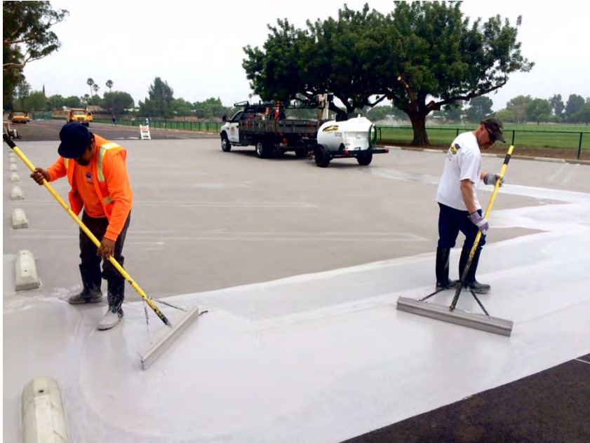
Two Coats of Guard Top Cool Seal are applied
