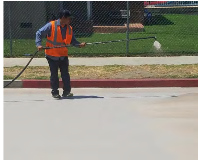
Second coat applied by hand spray
