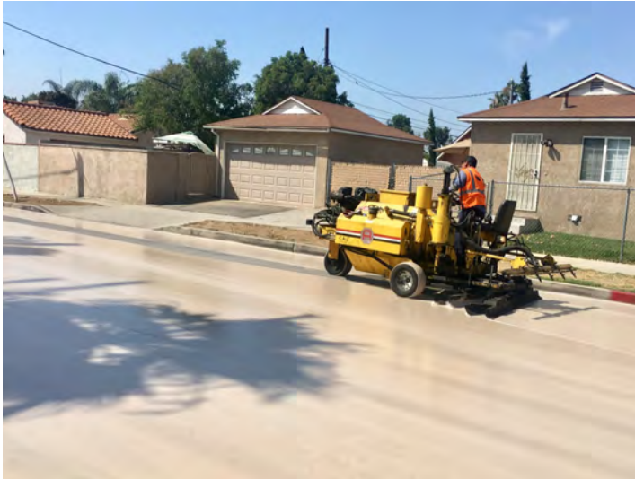
First coat applied using slurry buggy
