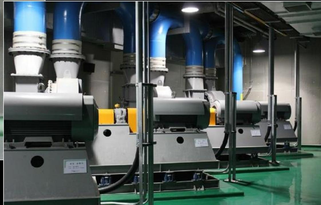
Garbage is extracted through under-ground vacuum tubes directly to an automated waste collection and processing plant.
