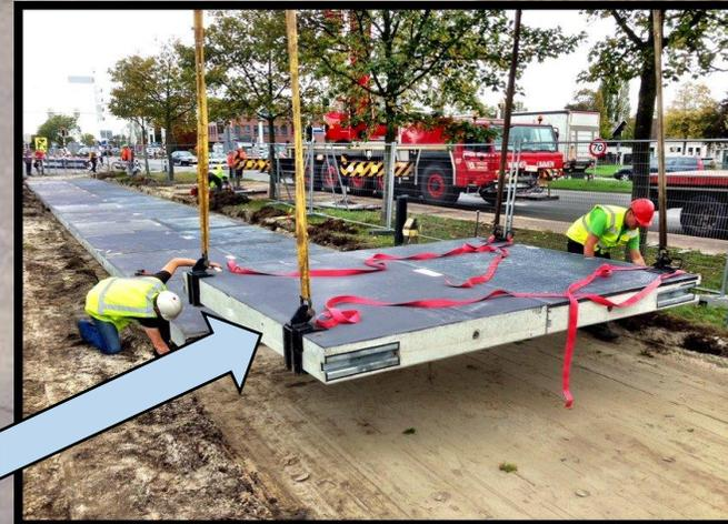
Solar cells imbedded in bikeway riding surface
